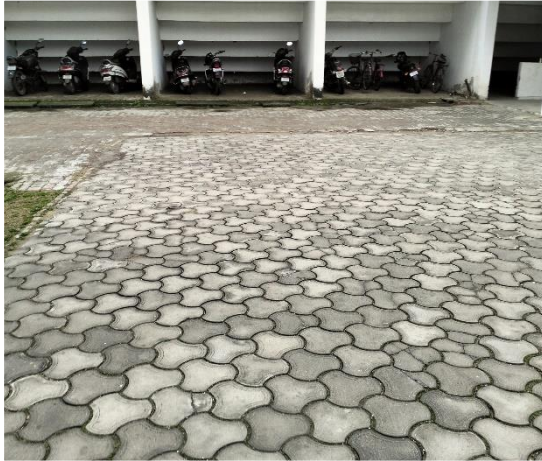
Paving stone installed in campus
