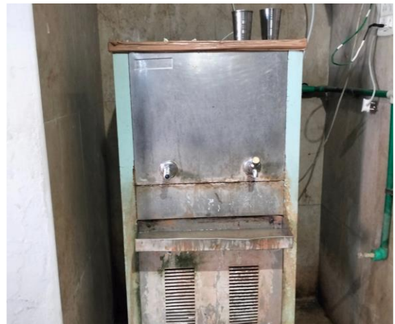
Push taps installed for water conservation
